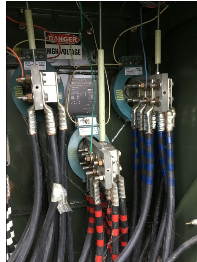
TYPICAL STACKED LUG INSTALLATION
